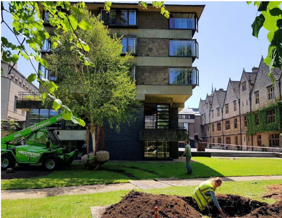
The root-balled silver birch, carefully being moved to its new location
