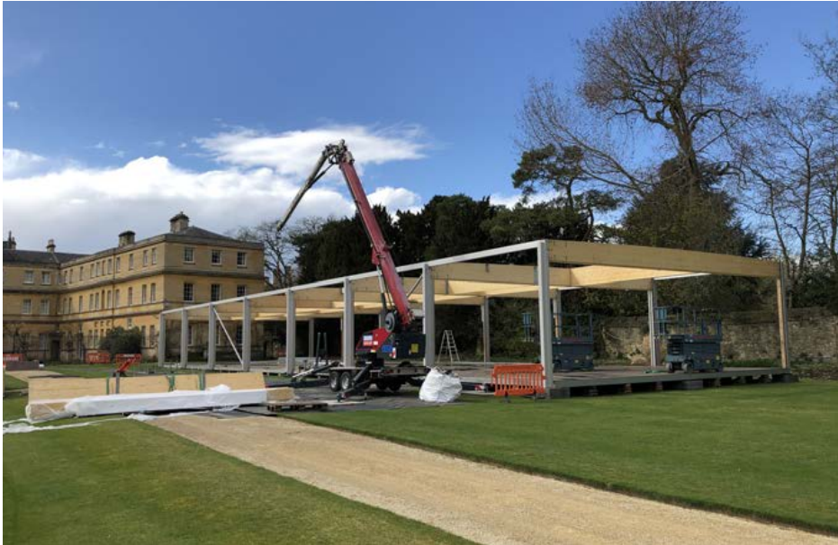
The Lawns Pavilion under construction
