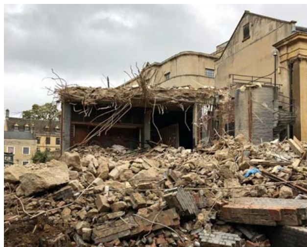
The demolition of Staircase 4
