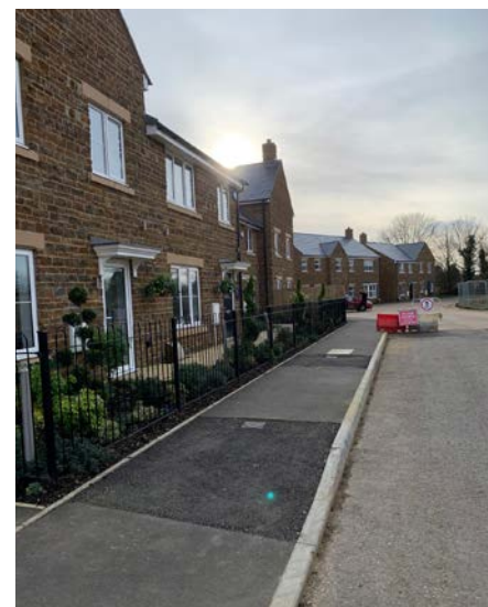
Housing at Drayton Lodge development
