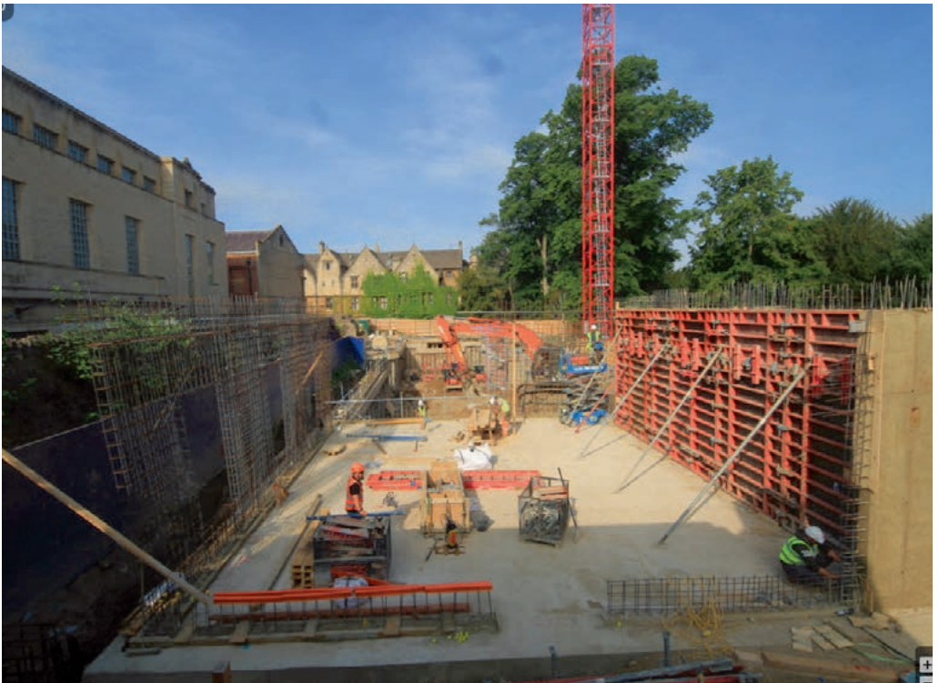
Construction of the Levine Building, June 2020
