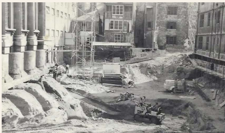
Excavating the former rose garden, which lay between the Jackson Building, to the right, and the library, to the left, to create the Norrington Room
