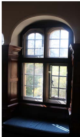
Below: secondary glazing has been installed in the Jackson Building
