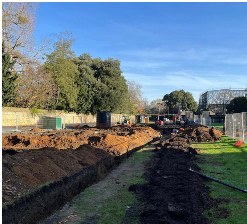
Trenches on the lawn during work to install ground source heat pumps
