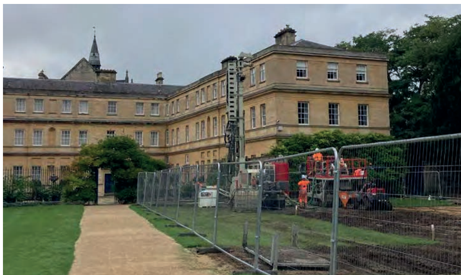
Immediately following the removal of the Lawns Pavilion, drilling machinery moved onto the Lawns for the installation of 22 boreholes to provide ground source heating for the Jackson Building
