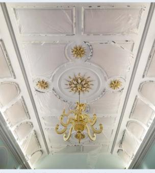
Above, the Hall ceiling with acoustic deadening panels (covered with protective sheeting), and the new colour on the walls; left, the servery area between the new kitchen and the Hall, which will have a glazed roof
