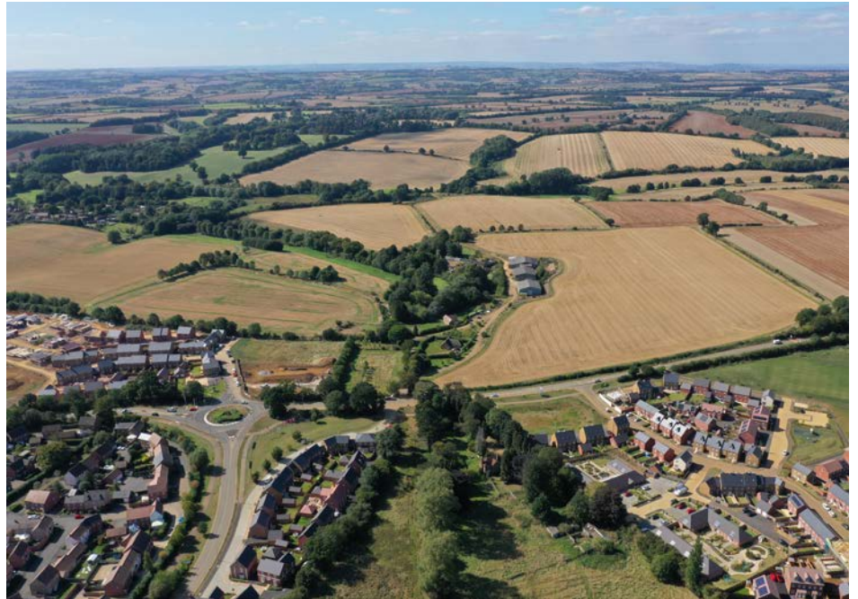
The Drayton Lodge housing development at Banbury
