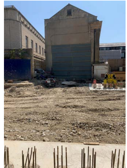
Demolition of the Cumberbatch Building ( above ), the archaeological survey in progress ( below left ), and the gable end of the library revealed, with the ring beam in the foreground ( below right )
