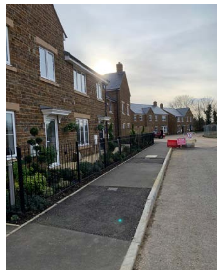
Housing at Drayton Lodge development
