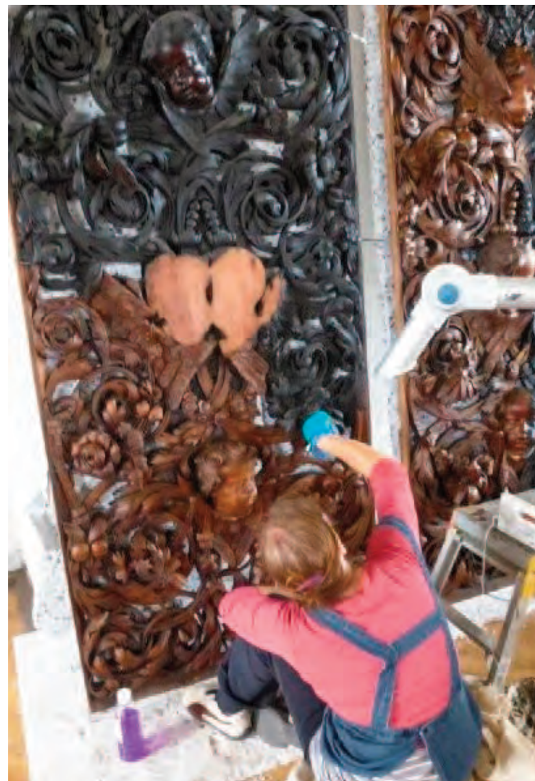
Dark stain being removed from one of the fretwork panels
