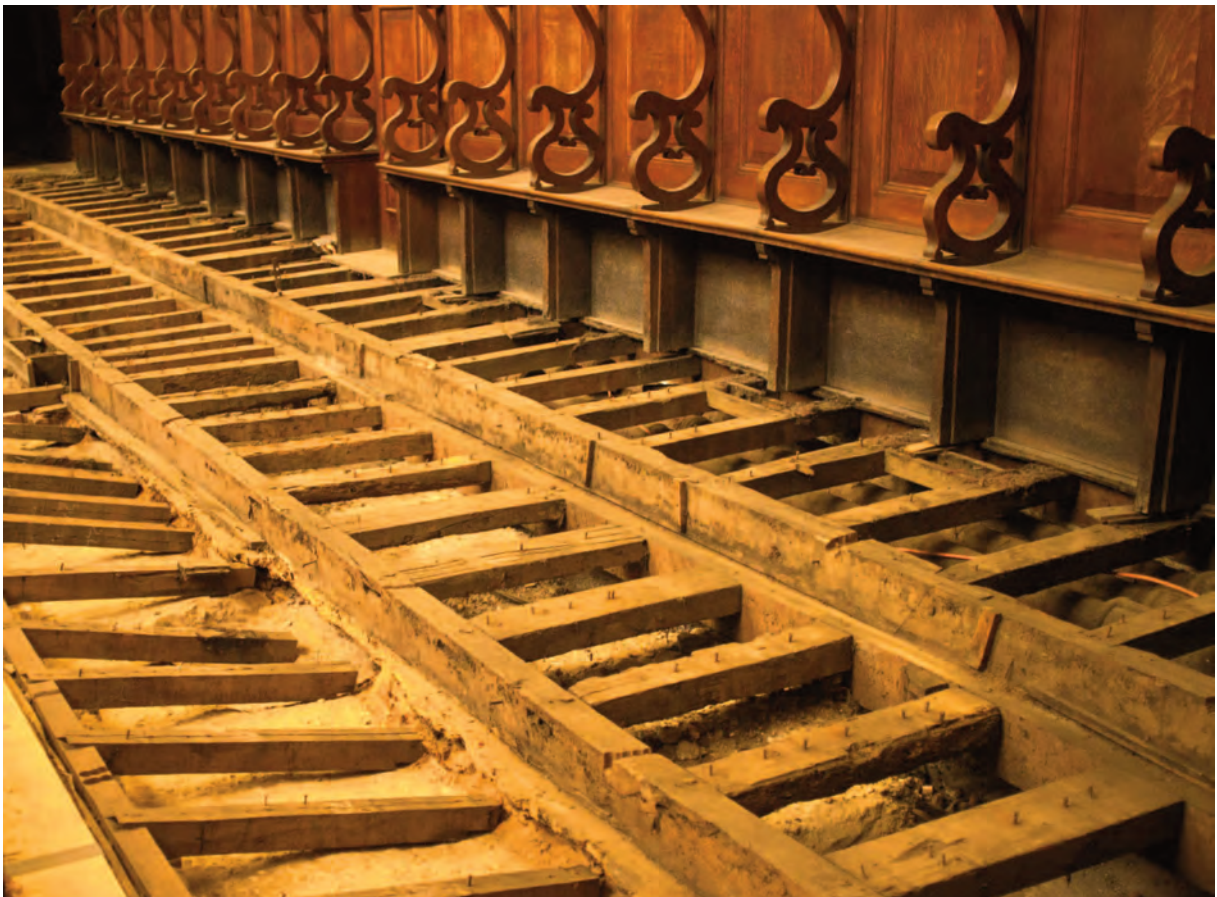
The pews flooring removed and the void cleaned, showing the collapsed lowest joists, which had been resting on pieces of brick and timber
