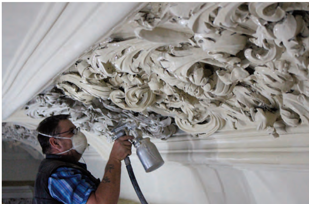
The cornice plasterwork being repainted
