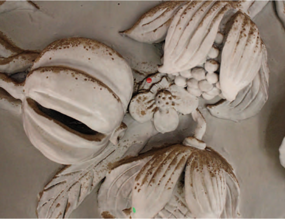
Detail of plasterwork, showing dirt and missing pieces (marked by coloured dots)
