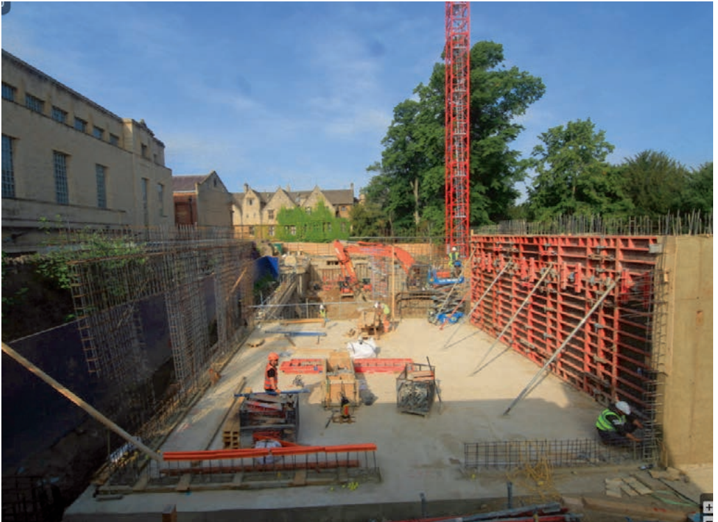
Construction of the Levine Building, June 2020
